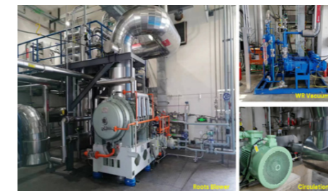
Electrification MVR upgrade project
